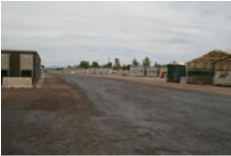
Figure 4 Treated roadway intersection. Product is visible during the 4-5 week maintenance phase
