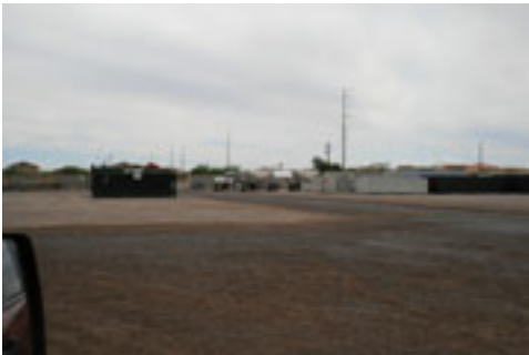
Figure 5 Treated Intersection after three weeks. Notice some track on but T.O.P. is still binding surface.
